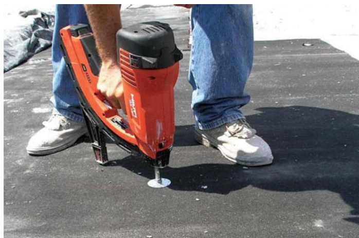
Figure 6. Fastening nonwoven geotextile fabric to existing concrete pavement
