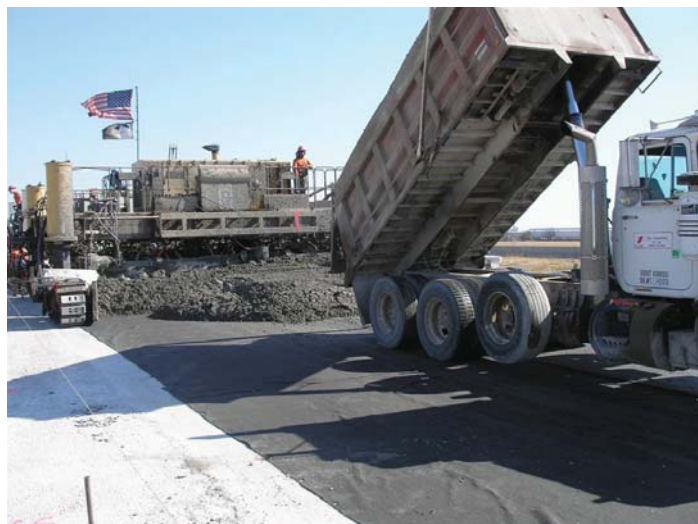
Figure 7. Paving on top of nonwoven geotextile materials
