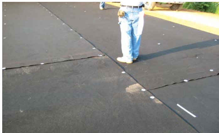
Figure 5. Overlap of nonwoven geotextile material sections
