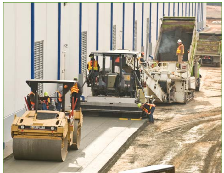
RCC paving train
