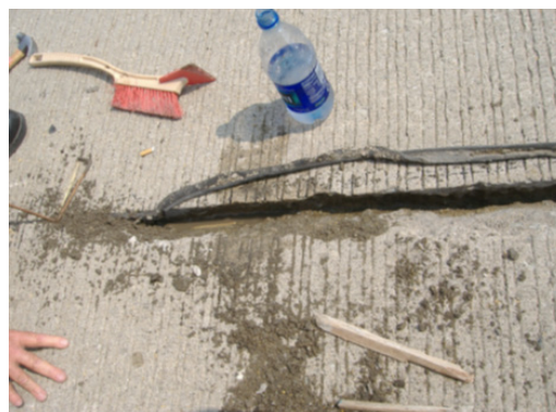
Figure 1: Typical examples of joint deterioration of concrete pavements in Indiana
