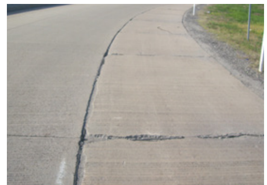
Figure 1: Typical examples of joint deterioration of concrete pavements in Indiana
