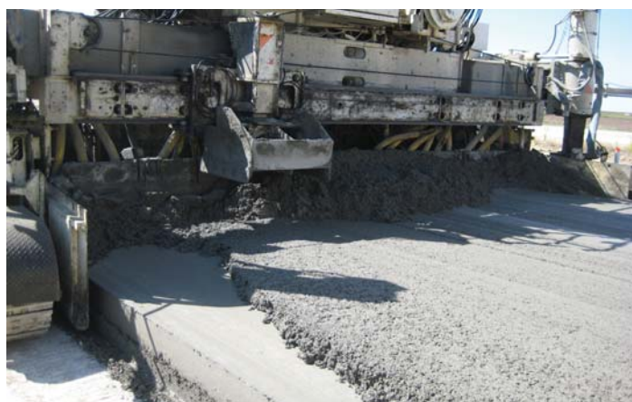
Two-lift concrete paving (courtesy of Kansas DOT)
