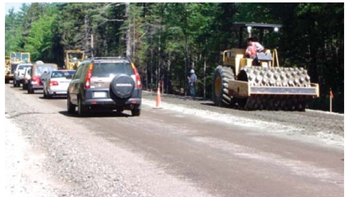
Figure 12. Traffic allowed on completed lane of full-depth reclamation prior to surfacing
