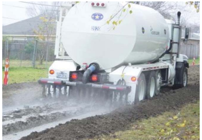
Figure 7. Placing cement in slurry form
