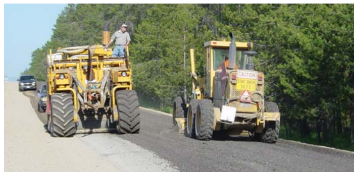
Figure 5. Reclaimer pulverizing existing asphalt and base material
