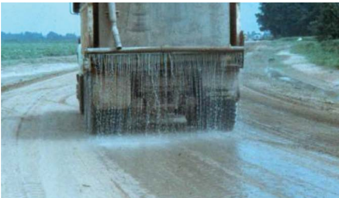
Figure 10. Water curing
