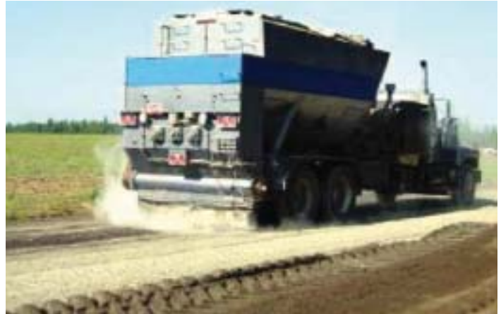
Figure 6. Placing cement in dry form
