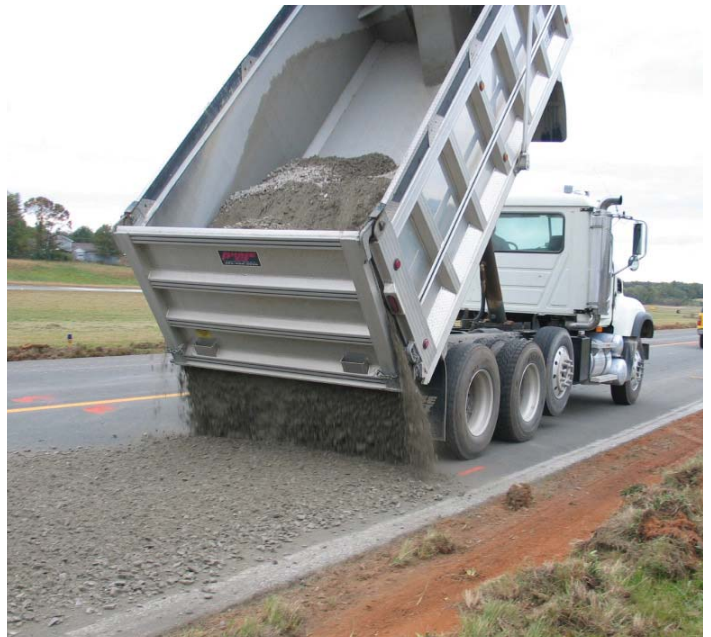
Figure 2. Placing additional aggregate prior to reclamation
