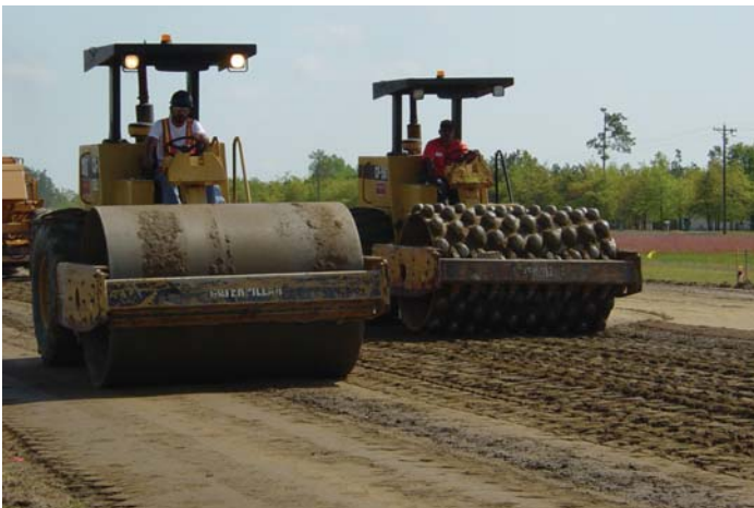
Figure 9. Compacting full-depth reclamation with vibratory and tamping rollers
