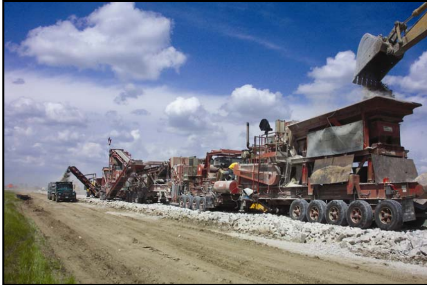
Figure 5. Paving trains recycle existing pavements in place
