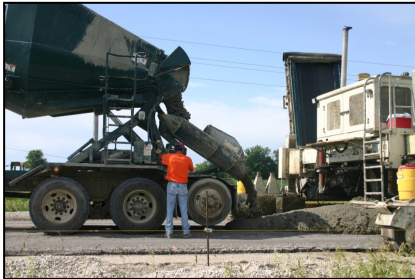
Figure 9. Concrete overlays can restore or enhance an existing pavement's functional and structural performance
